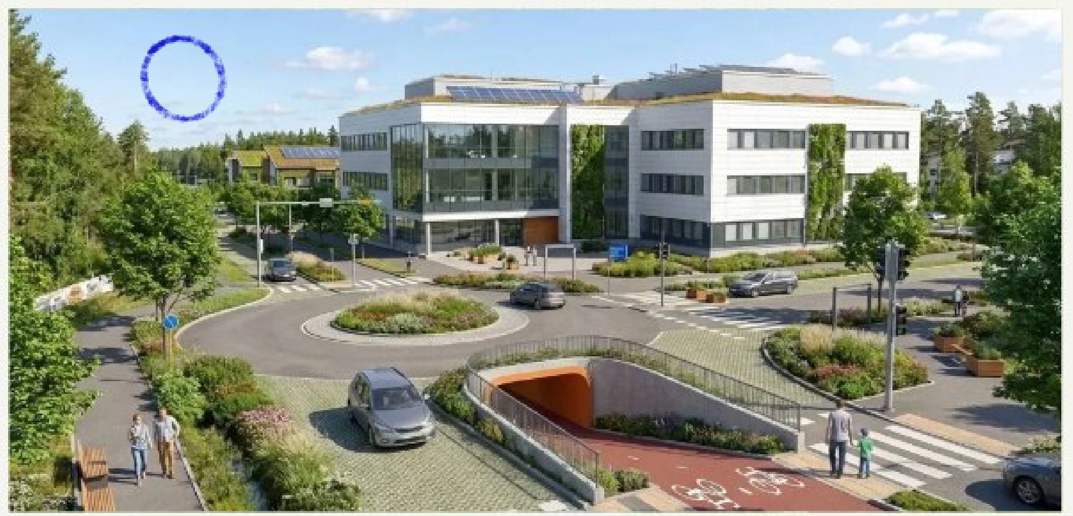
Green Roundabout with Cyclist Tunnel A roundabout with greenery to create a friendly environment. A tunnel separates cyclists from traffic, while elements such as curved paths and planted islands naturally slow drivers. The result is a safer, calmer, and more inviting gateway to the school, trotting track, and tram stop.
